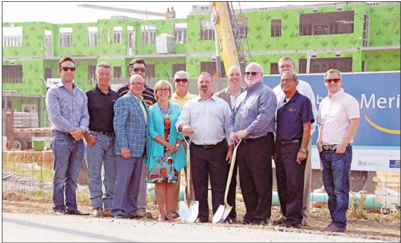
Piroli Group Developments president Rob Piroli and Leamington mayor John Paterson (seventh and ninth from left, respectively) hold ceremonial shovels while surrounded by associates and partners for the Seacliff Heights project Friday, Aug. 28. The groundbreaking ceremony took place about five months after construction for Phase 1 began because of building permit delays.
